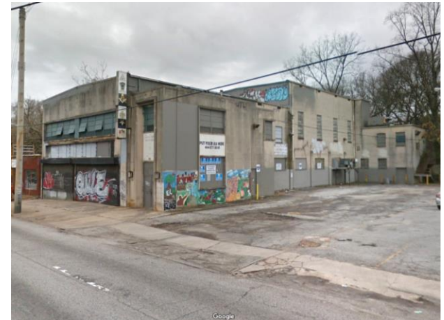
Masonic Building – Current Condition
